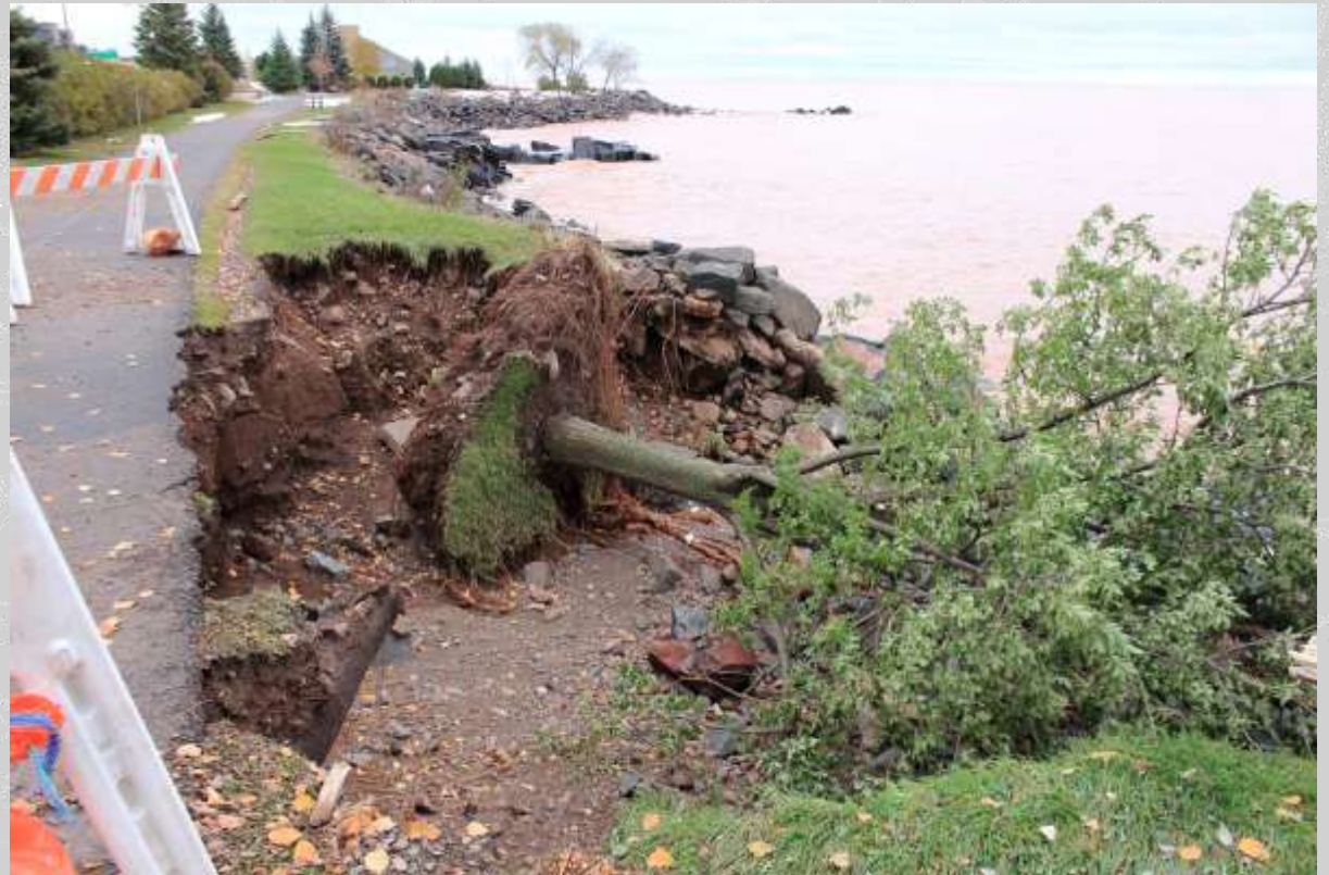
Erosion from the waves along Duluth's lake walk Photo credit Ken Slatten
