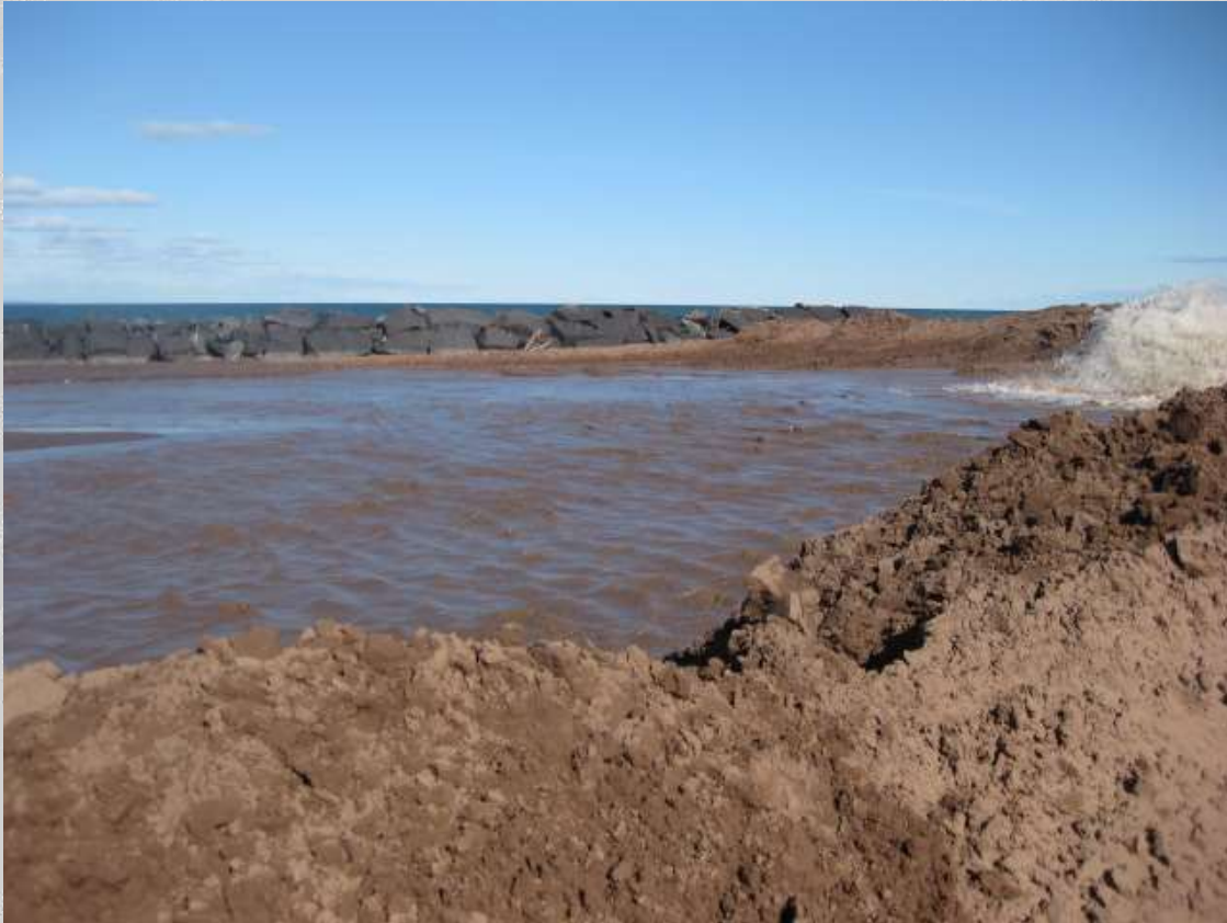
Dredged material placed near Superior Entry NW Breakwater, Photo credit DuAO, 10/2008
